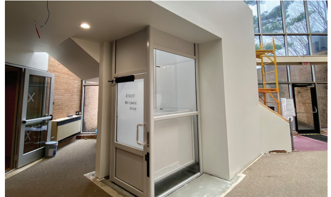
New ADA Accessible Elevator Lift to second floor and municipal court.
