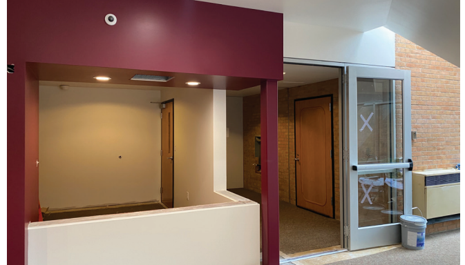
New reception area for residents adjacent to the Police Department.
